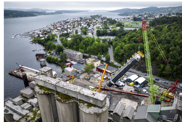
Brevik CCS facility in Brevik, Norway. Image courtesy of SLB Capturi.
