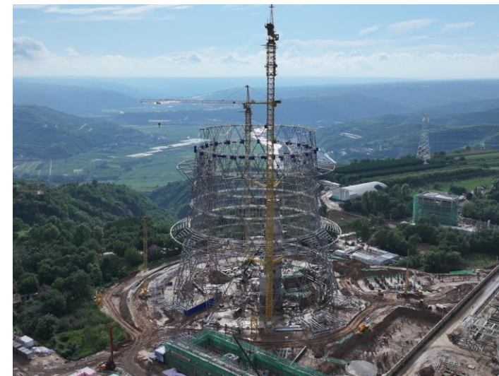
Huaneng Longdong CCUS project under construction. Image courtesy Huaneng Clean Energy Research Institute.
