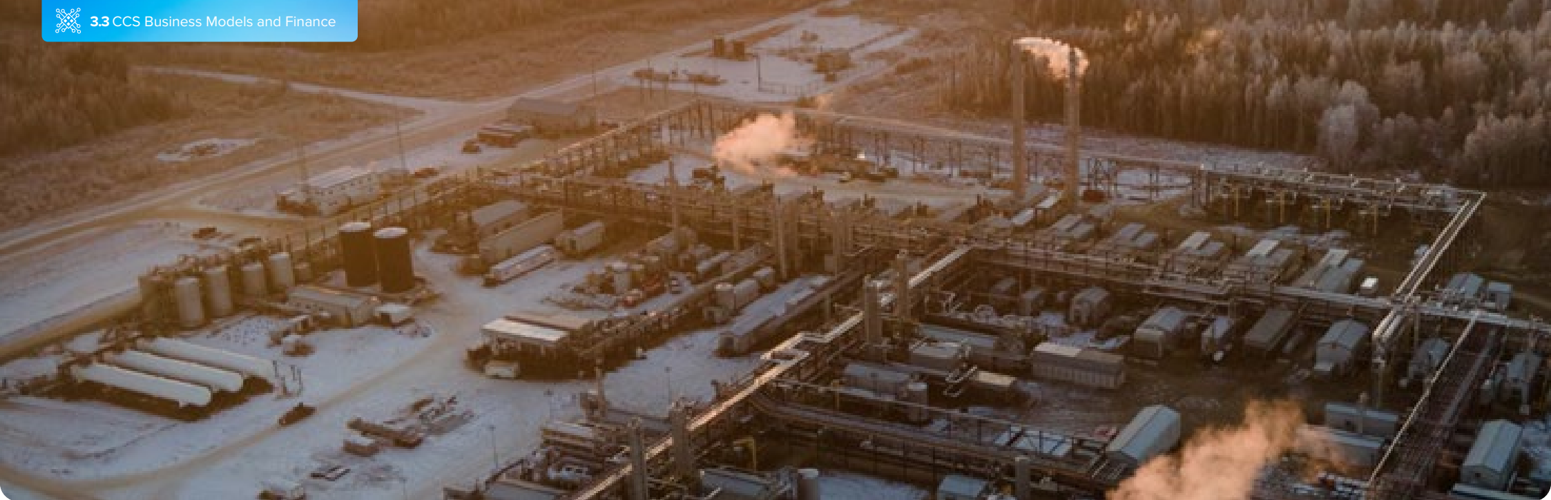
Advantage Glacier Gas Processing Facility with Entropy's Integrated (iCCS™) and Modular (MCCS™) Carbon Capture Technology in Canada. Image Courtesy of Entropy Inc.
