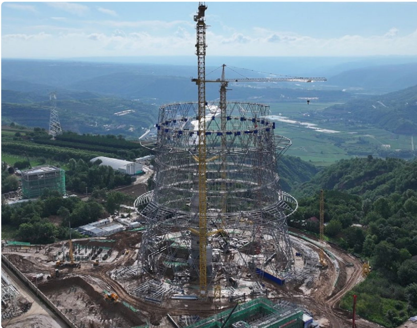
Huaneng Longdong CCUS project under construction, image courtesy Huaneng Clean Energy Research Institute
