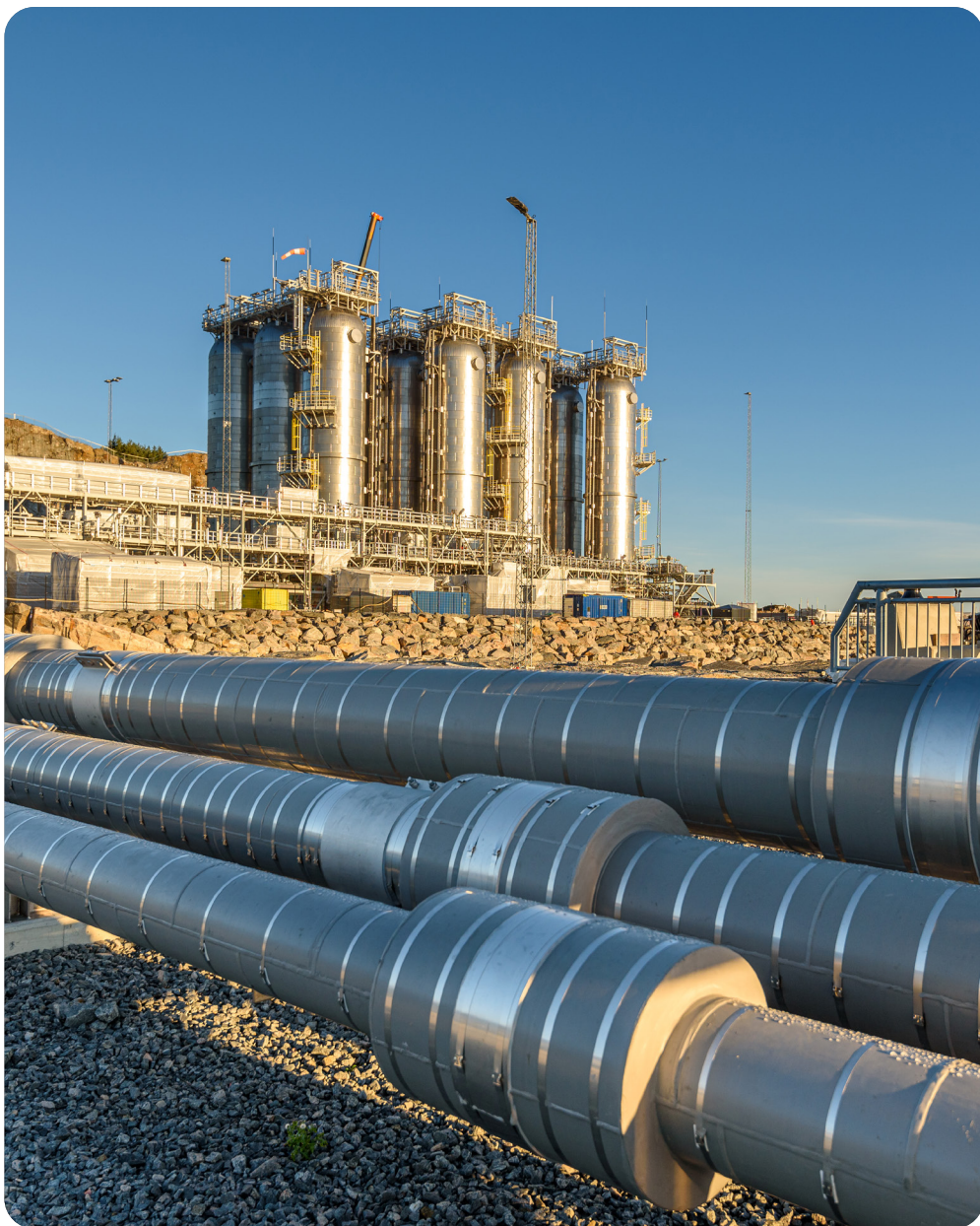
Northern Lights onshore pipeline, Norway. Image courtesy Northern Lights JV.
