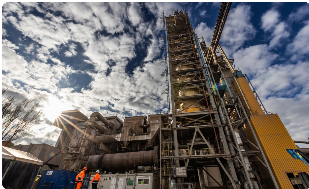
Leilac-1 Pilot Plant at the Heidelberg Materials Plant in Lixhe, Belgium. Image courtesy of Leilac Ltd.
