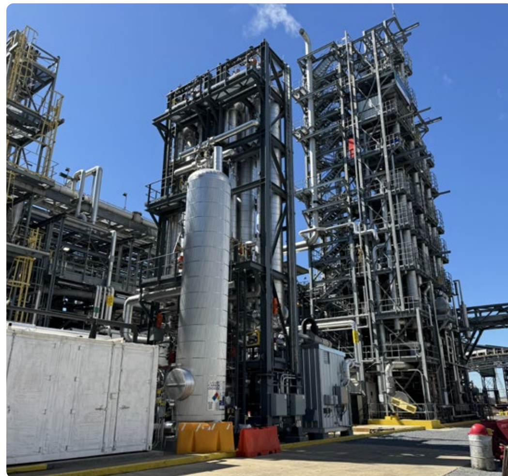
Carbon America's FrostCC™ pilot at the National Carbon Capture Center in the US. Image courtesy of Carbon America.
