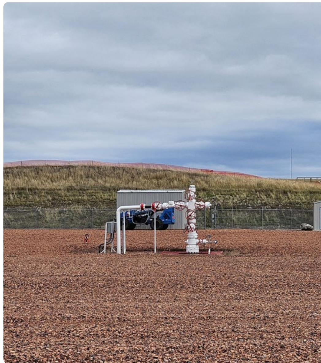
A CO 2 injection well at the Dakota Gasification CO 2 sequestration site near Beulah, North Dakota. Image courtesy Dakota Gasification Company.
