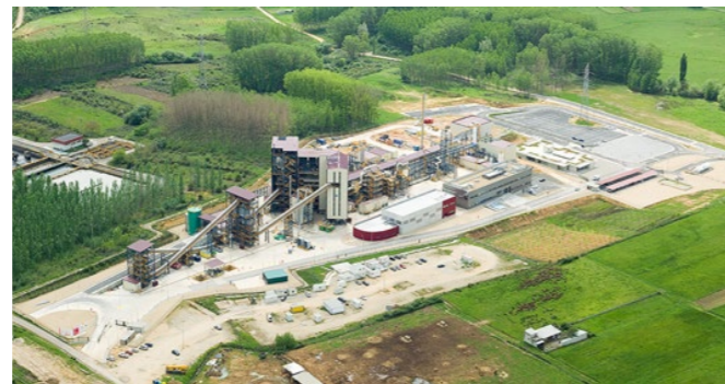
30 MWth SFW Oxy+ plant in Ponferrada, Spain: Carbon capture and storage demonstration plant with Endesa and CIUDEN during 2009-2017. Design for a full scale 300 MWe plant was developed as part of the project.
