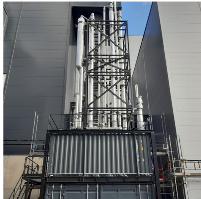
Sumitomo SHI FW (SFW), together with partner Capsol Technologies ASA, and Swedish energy company Växjö Energi AB collaborate on a testing campaign to demonstrate carbon capture technology based on the hot potassium carbonate (HPC) process.
